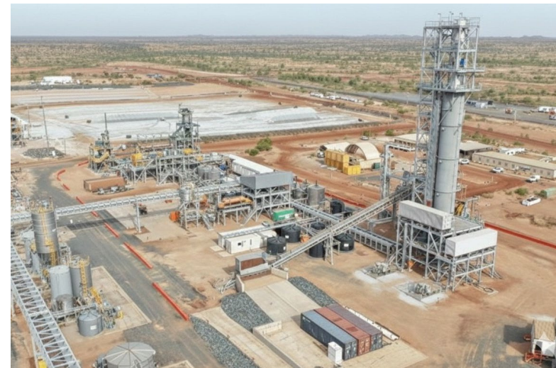
Constructed Mid-Stream Demonstration Plant with Pilbara Minerals – Pilgangoora, Pilbara, WA
