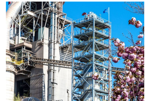
Leilac-1 pilot plant built 2019 at Heidelberg Materials cement plant – Lixhe, Belgium
