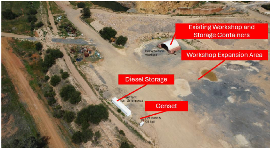
Figure A22: Existing mining and diesel power infrastructure at Mt Boppy.
