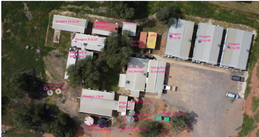
Figure A21: Existing camp facilities located at Mt Boppy.
