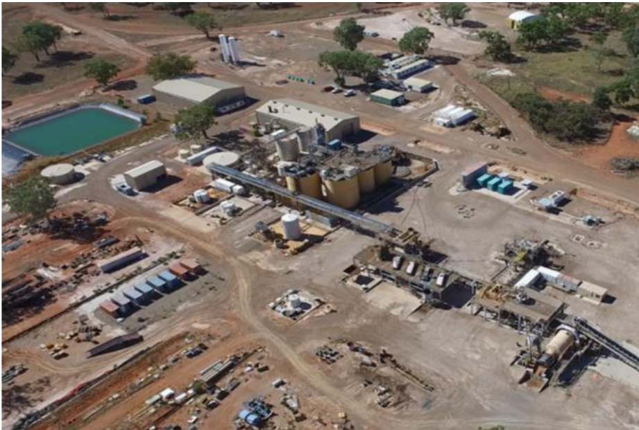
Figure 3: The existing Wonawinta Processing Plant.
