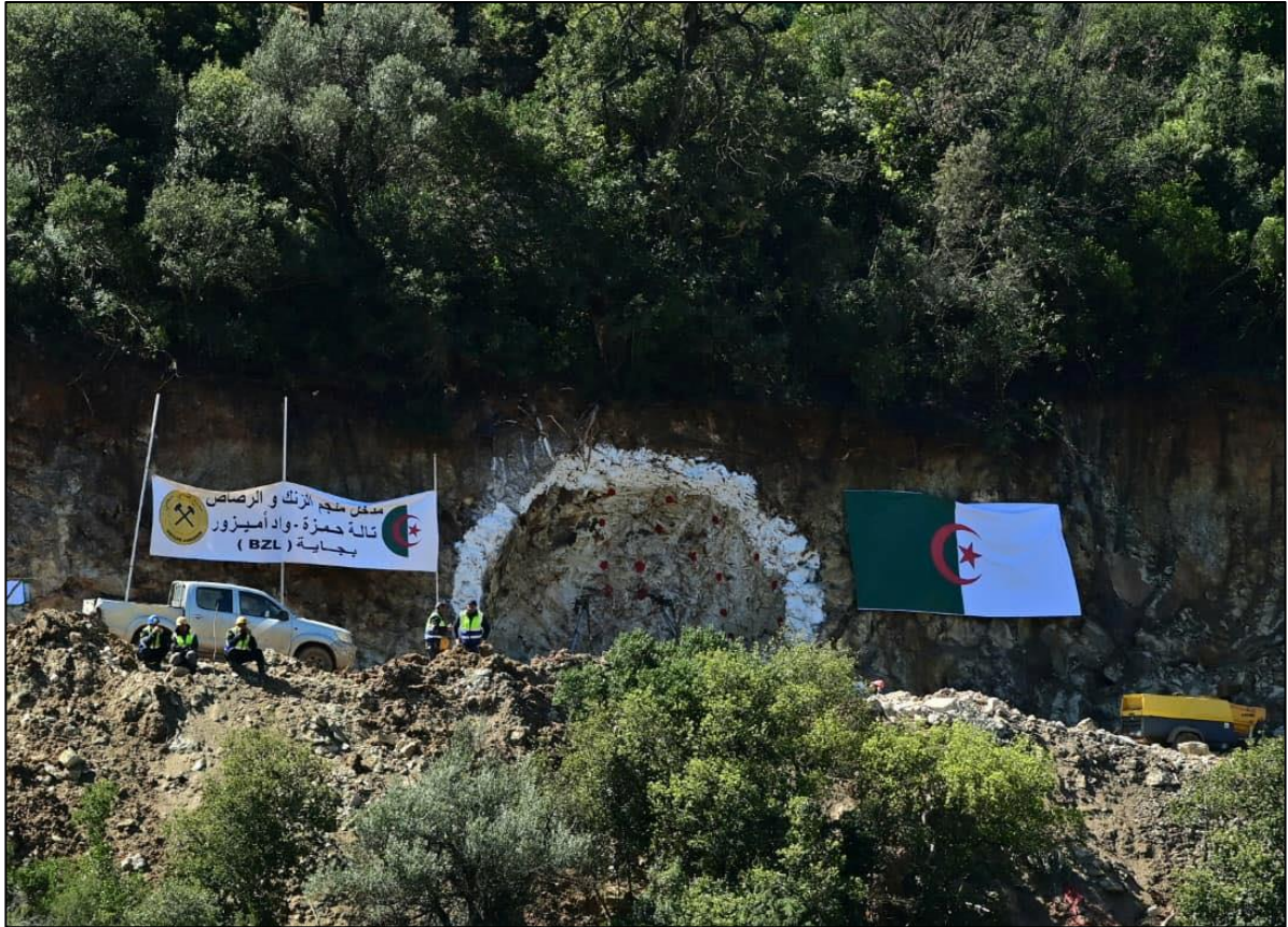
Figure 2: Early access works at site of the portal
