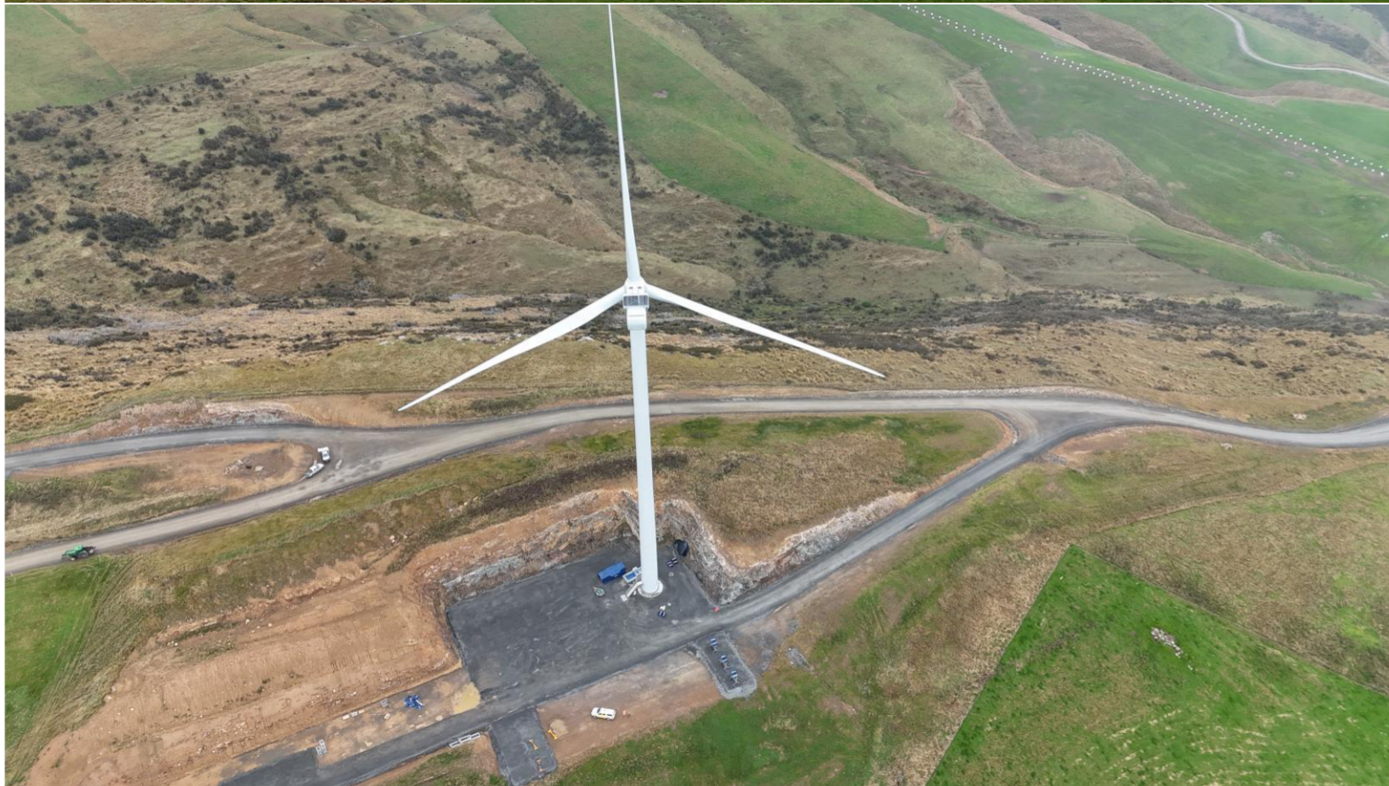
Kaiwera Downs Stage 2 under construction
