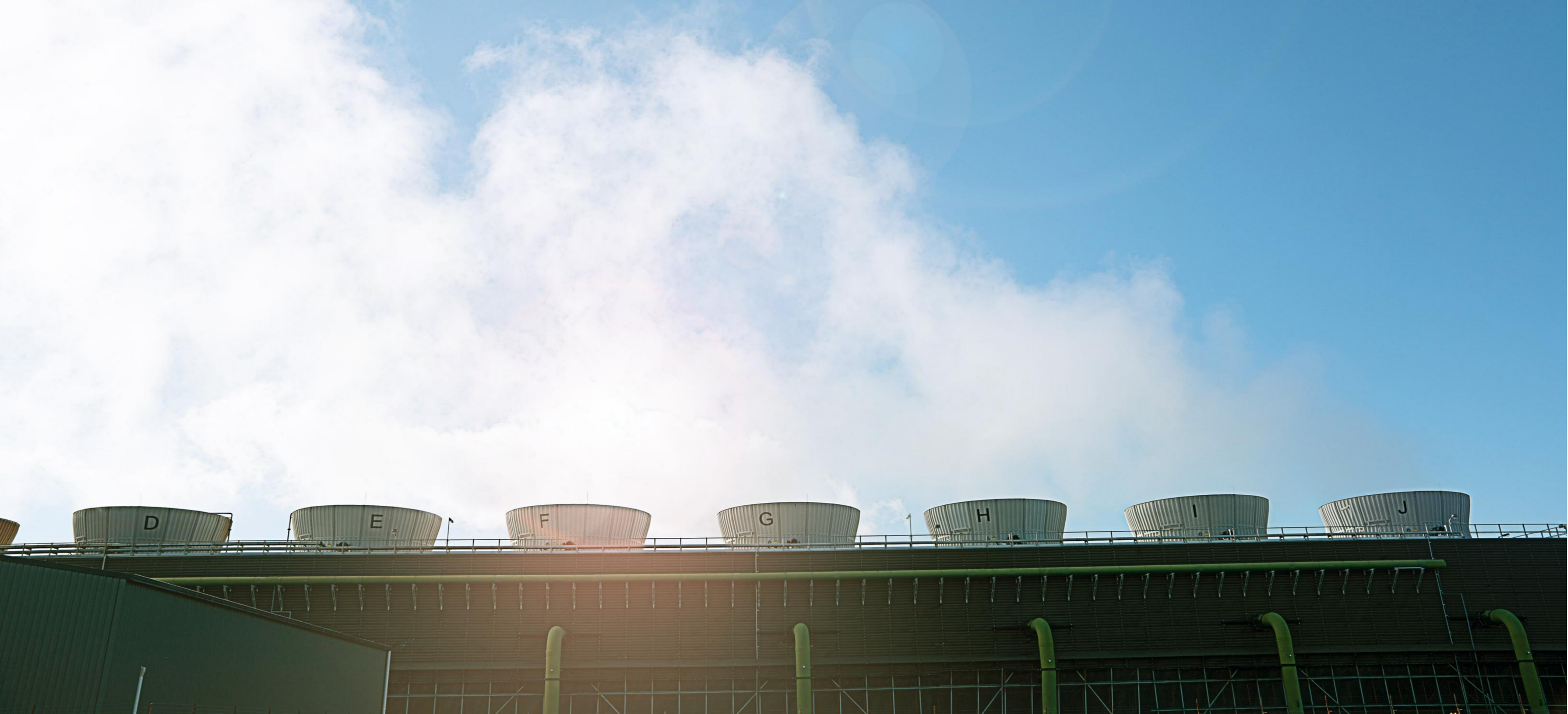
Ngā Awa Pūrua cooling tower
