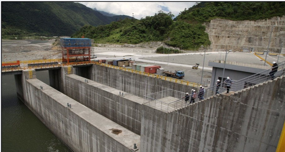
Coca Codo Sinclair hydroelectric power plant, operating since 2016
