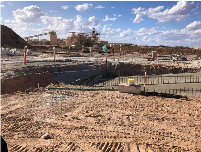
Figure 5: Wash plant pad and sumps.
