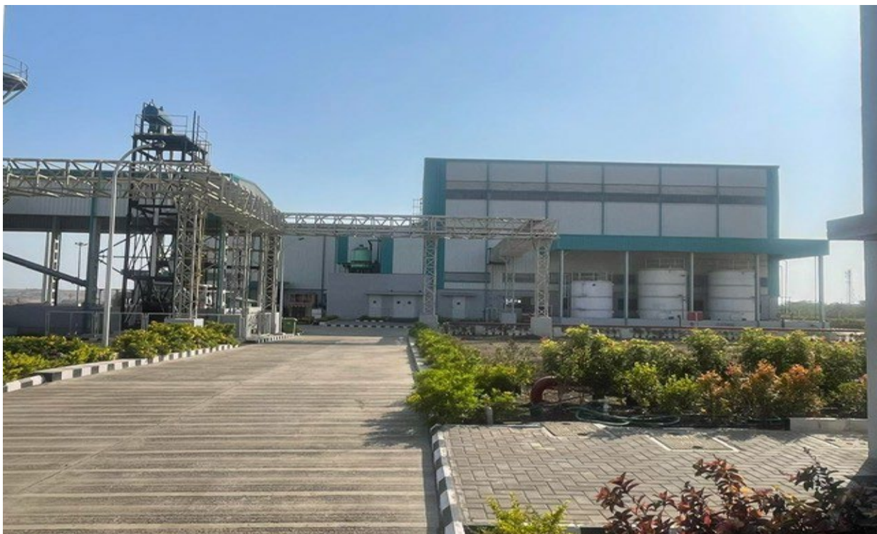
Our Expandable Graphite JV Facility near Pune, India
