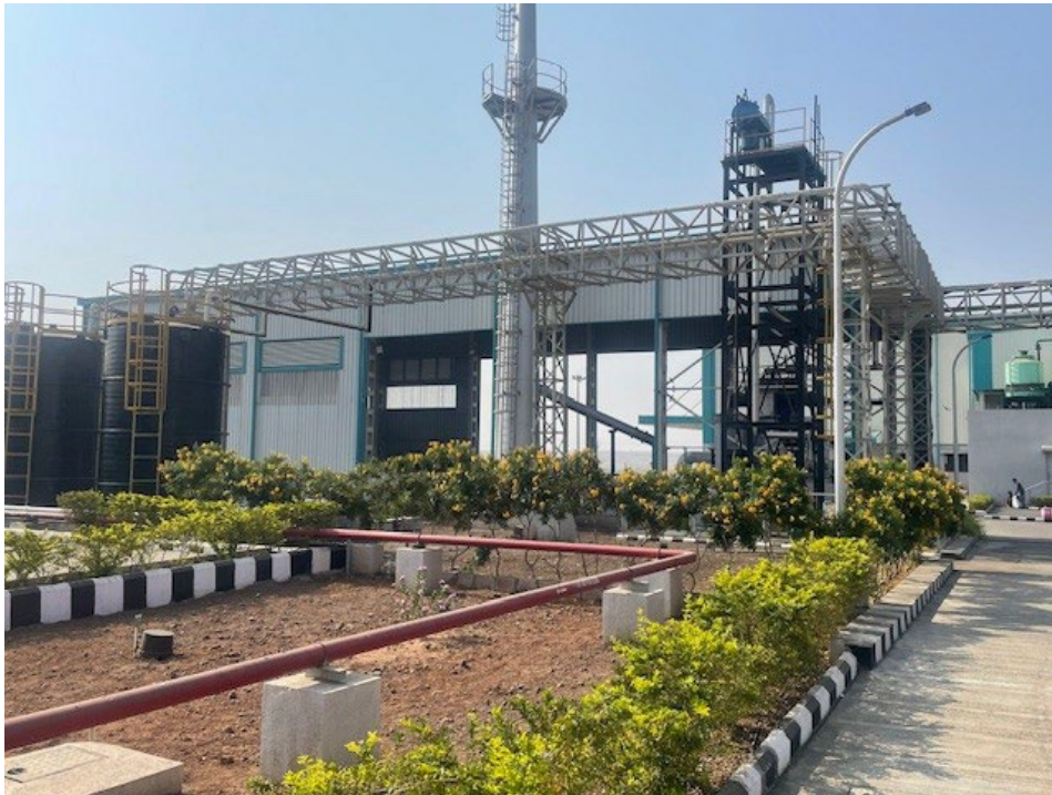
Figure 1 – Part of the expanded facility at PGT
