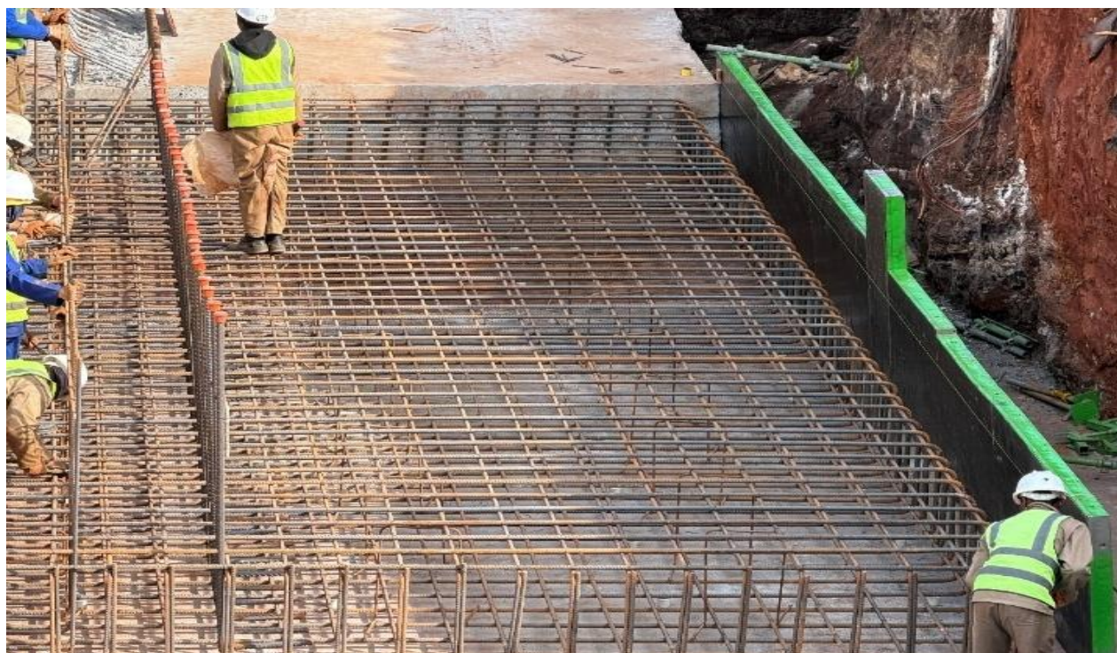
Figure 4: Retaining wall foundation steelworks
