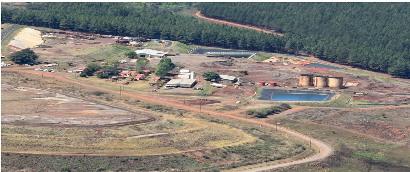
Figure 11: Aerial photo of the existing Plant post decommissioning of old facilities.
