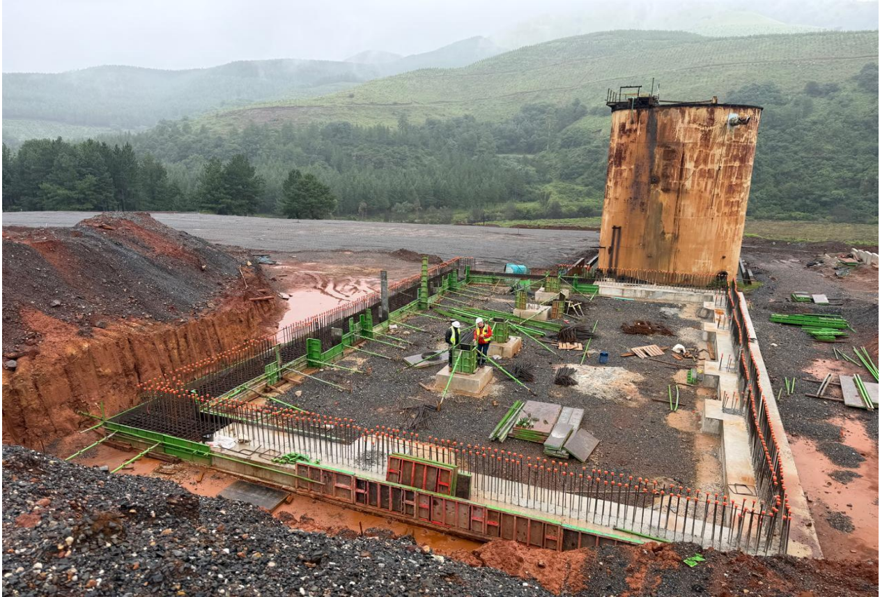
Figure 2: Civil works underway for Gold Room foundations.
