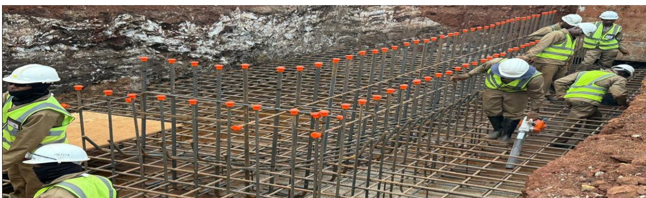
Figure 9: Steel reinforcing installation and preparation for concrete placement
