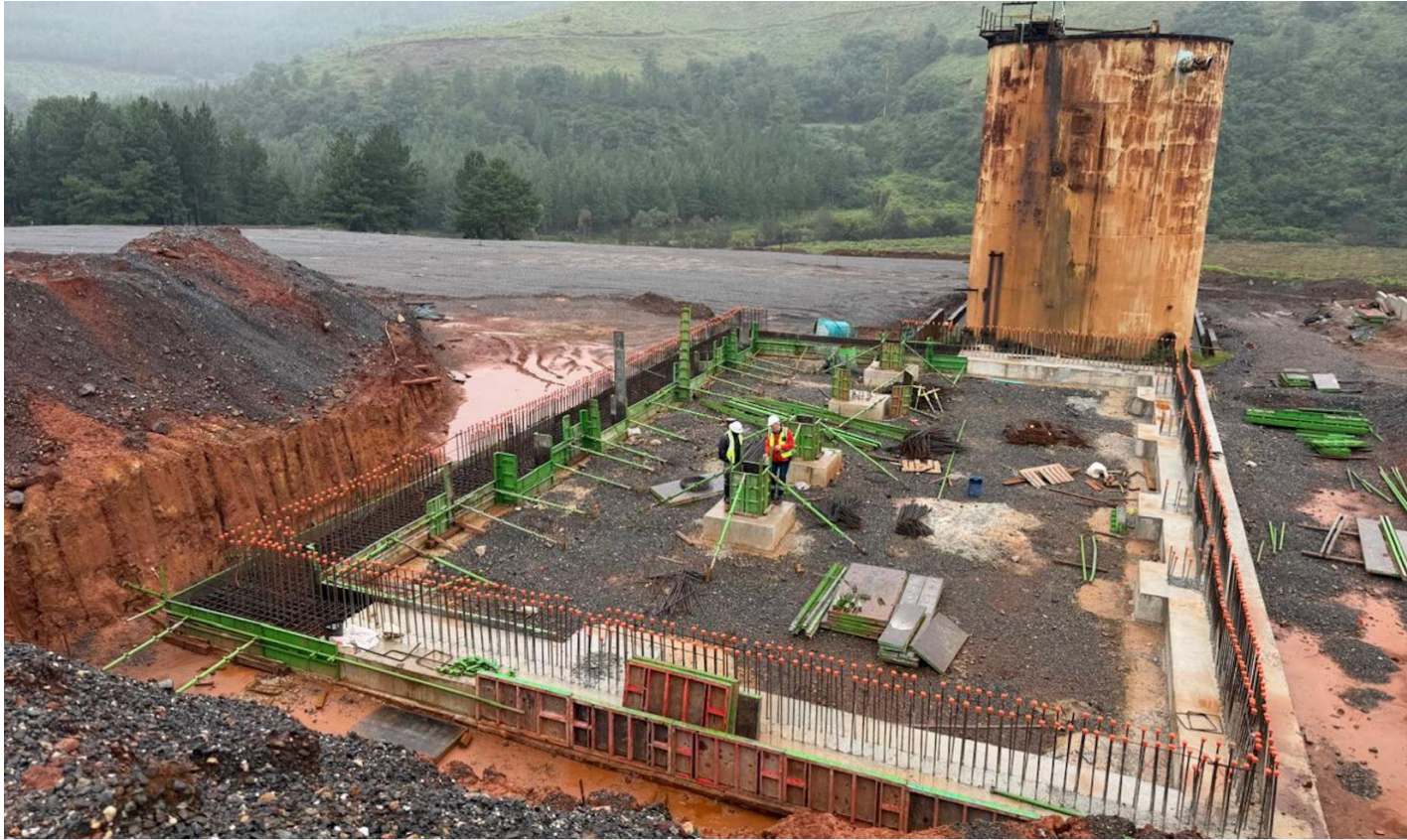
Figure 10: The Gold Room's Foundations
