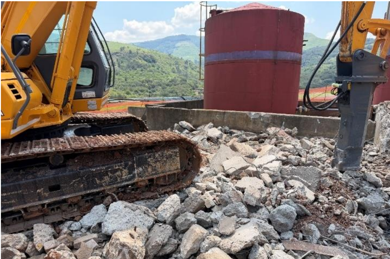
Figure 3: Removing old engineering structures
