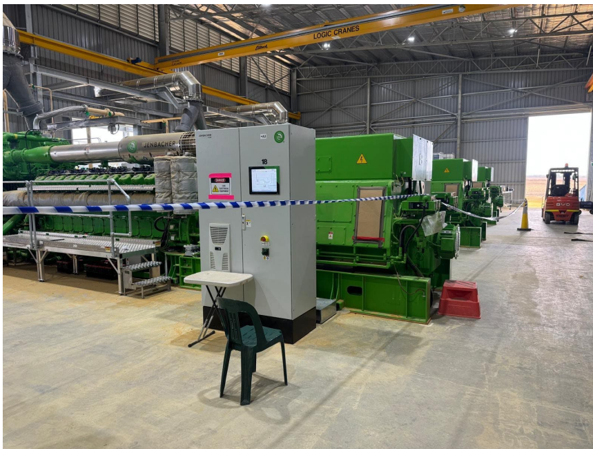
Pre-Commissioning Generator Energisation
