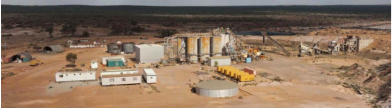
Figure 7: Aerial view of Plant before re-location.
