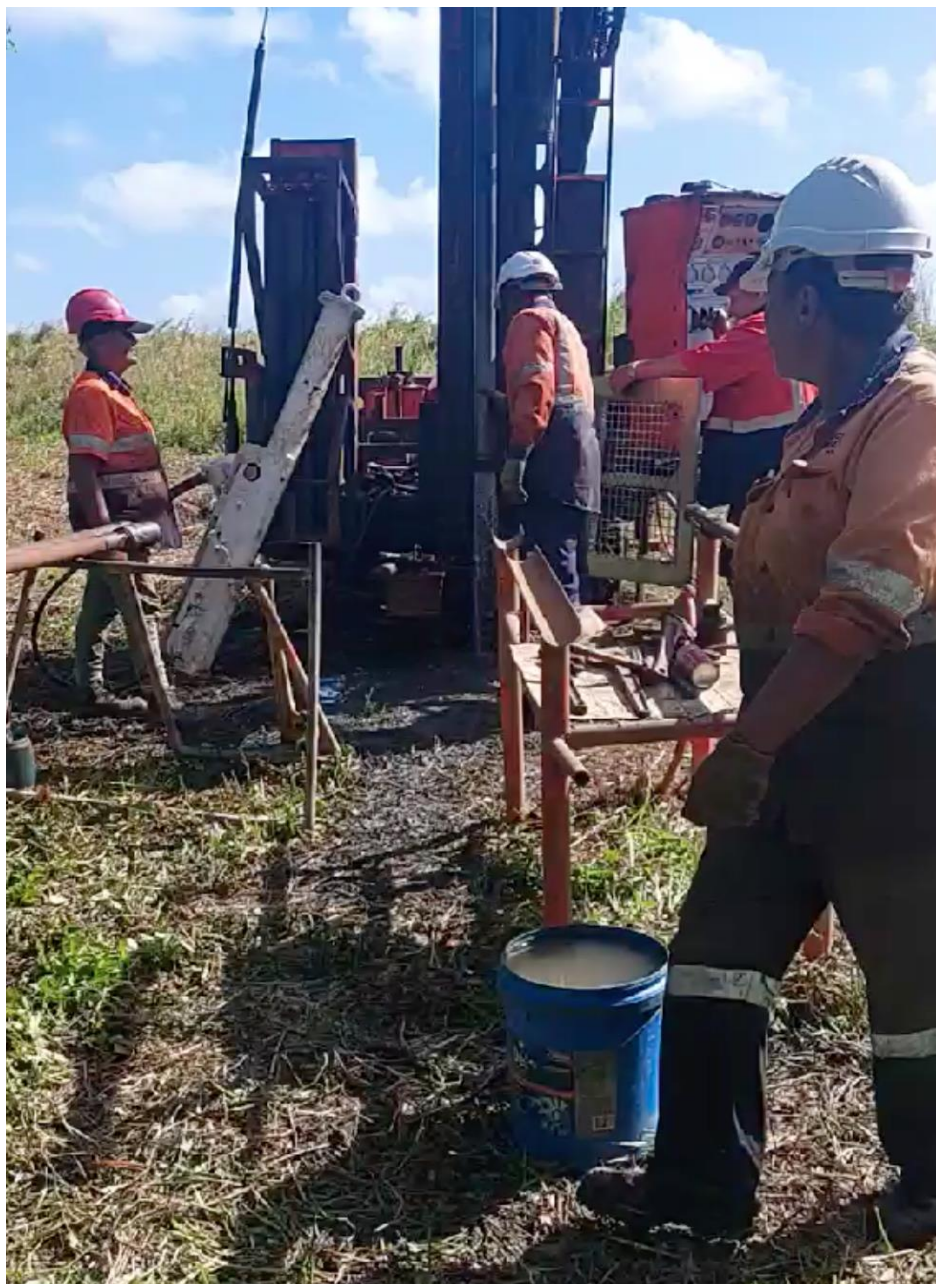
Plate 6 – Geotech drilling program at Kulukulu South sand processing plant site
