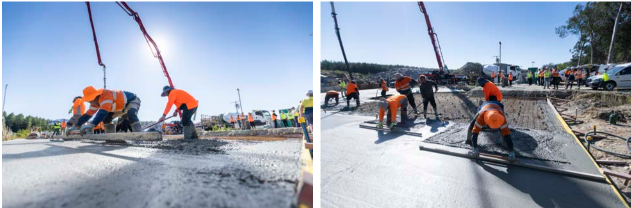
Figure 1: Finishing Work at the AusPozz™ Commercial-Scale Concrete Demonstration Pour
