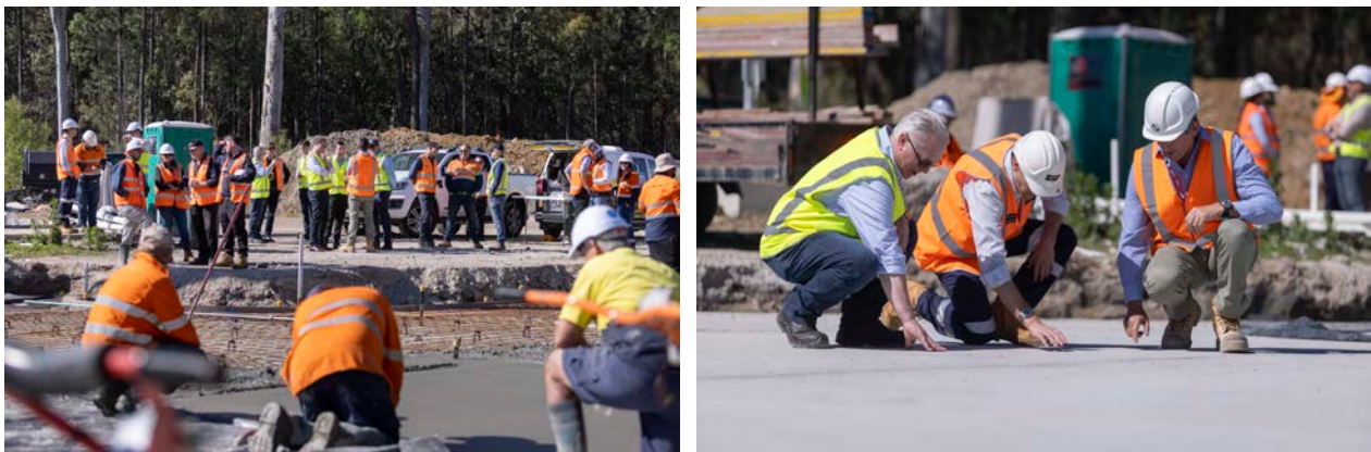
Figure 2: Attendees at the AusPozz™ Commercial-Scale Concrete Demonstration Pour
