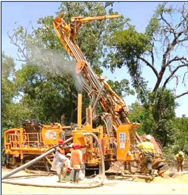
Figure 4 | RC drilling in September quarter at Ferke
