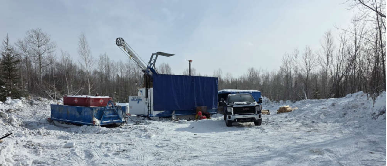
Figure 2 – Drill rig set-up at the Rouyn Gold Project – Astoria Project Area, Québec.
