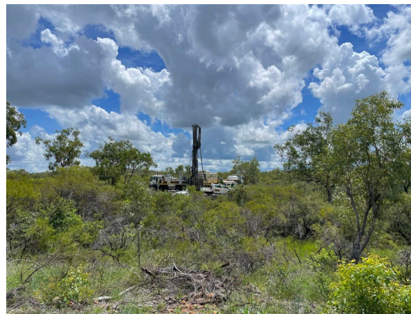
Figure 14: RC drill rig set up on Hole 24RCDH11
