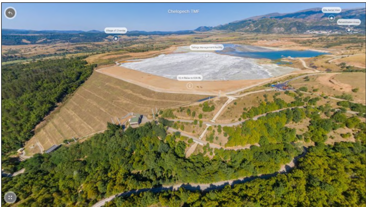
FIGURE 18-2: TAILINGS MANAGEMENT FACILITY
