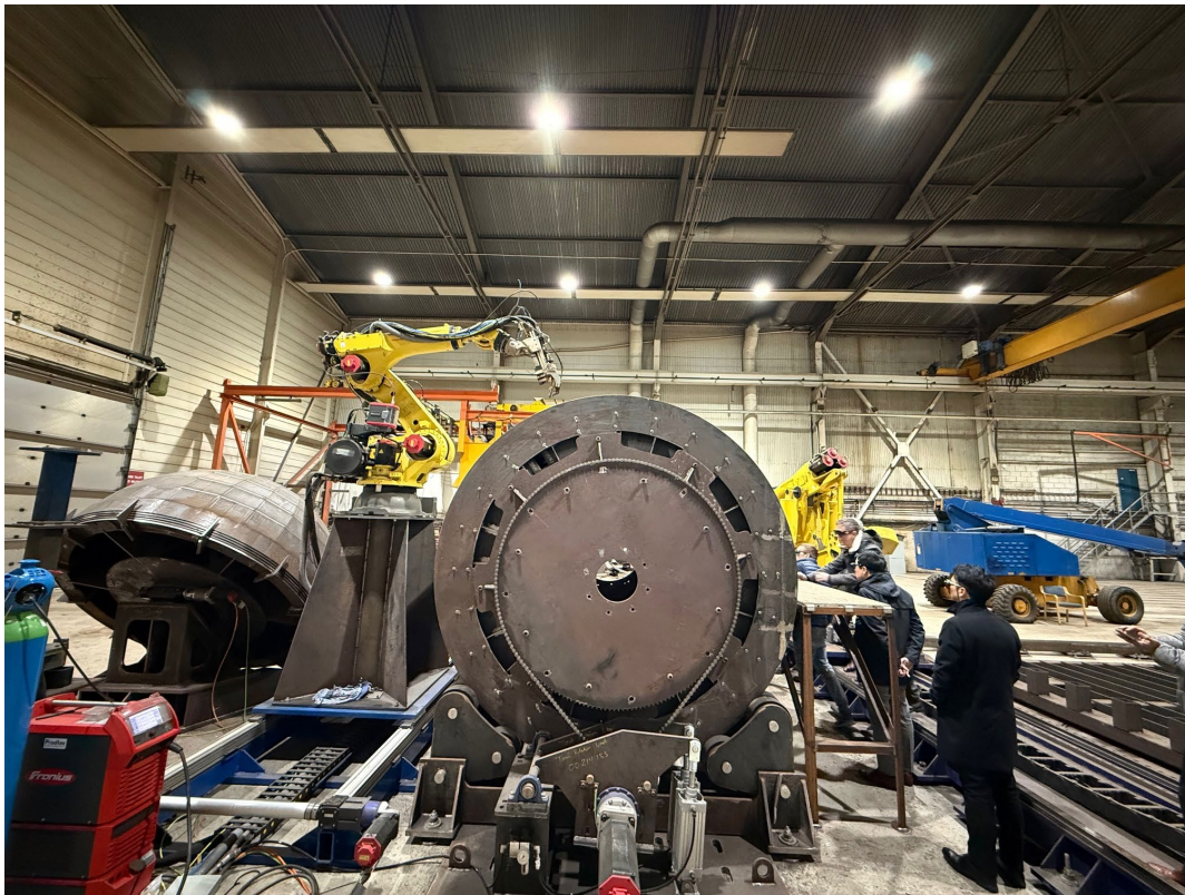
Robotic Cell: Cylinder and End-Cap Jigs with hydraulics to rotate tank
