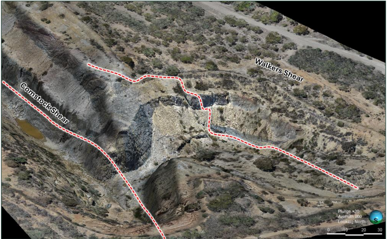
Figure 5 – View of the high-accuracy LiDAR and photogrammetry of the southern end of the Comstock open-cut with key projected structures – looking towards the North (azimuth 000). Entrance to the pit is currently possible from the Southeast.
