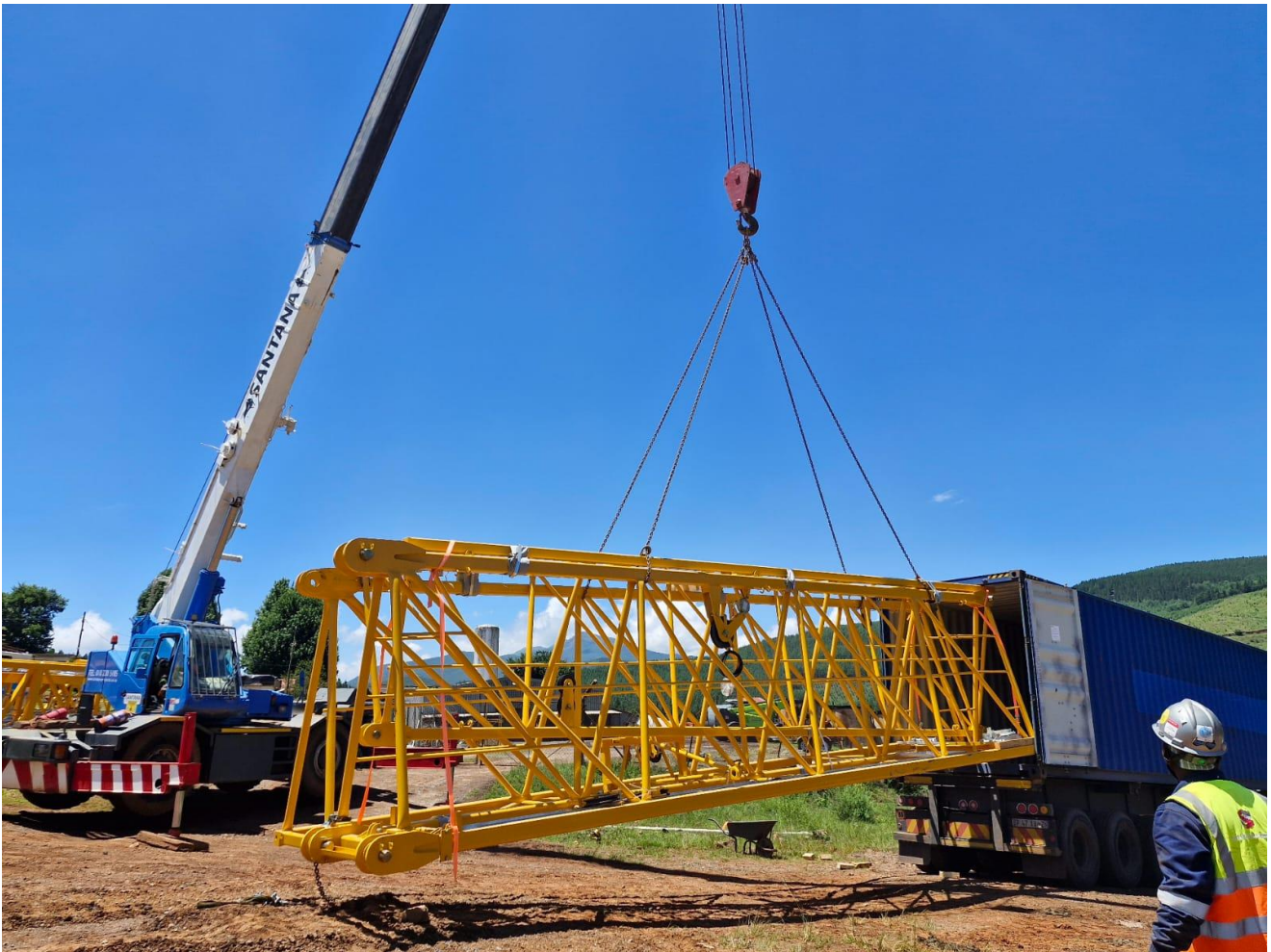
Figure 3: Tower Crane delivered to site
