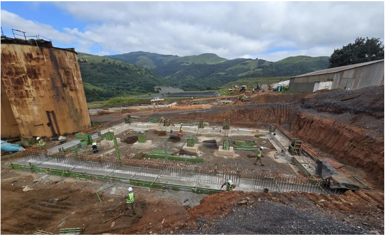
Figure 2: Plant construction underway
