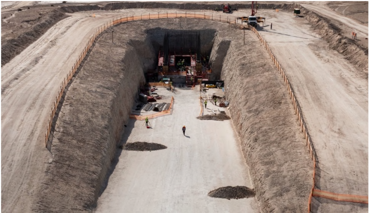
Figure 2: The first concrete pour at the primary crusher site has been completed. A total of 500m 3 was poured at an average flow rate of 40m 3 per hour.
