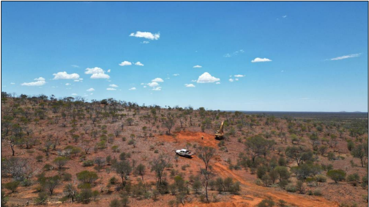
Figure 2: Drill pad preparation at Mt Kersey
