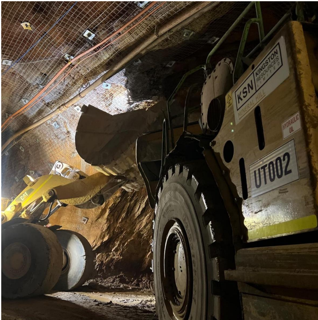
Figure: Underground development underway
