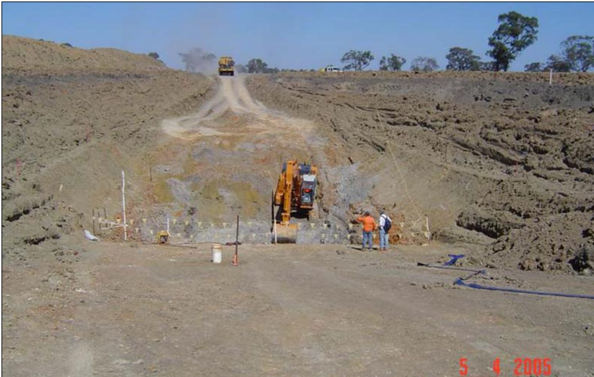
Figure 16.4 Test pit excavation viewed from northern end
