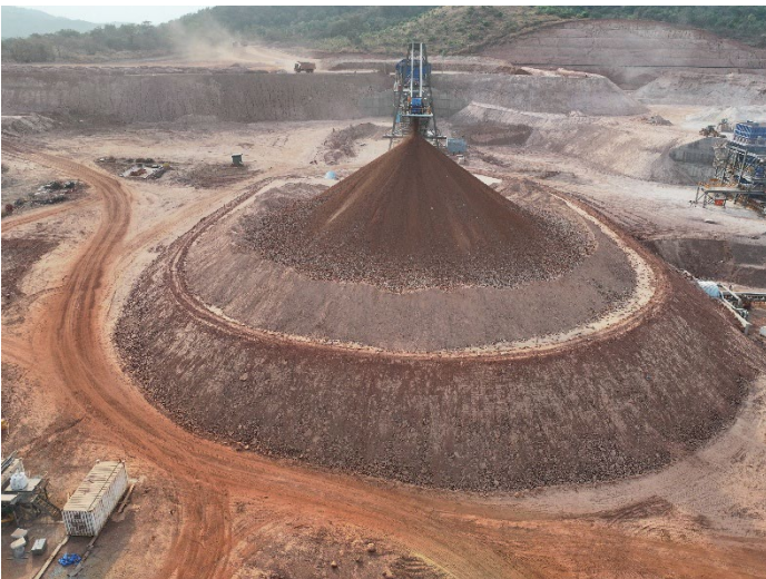
Figure 3: Primary Crusher – Ore Reclaim Feed
