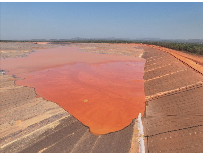
Figure 5: Tailings Facility Storage
