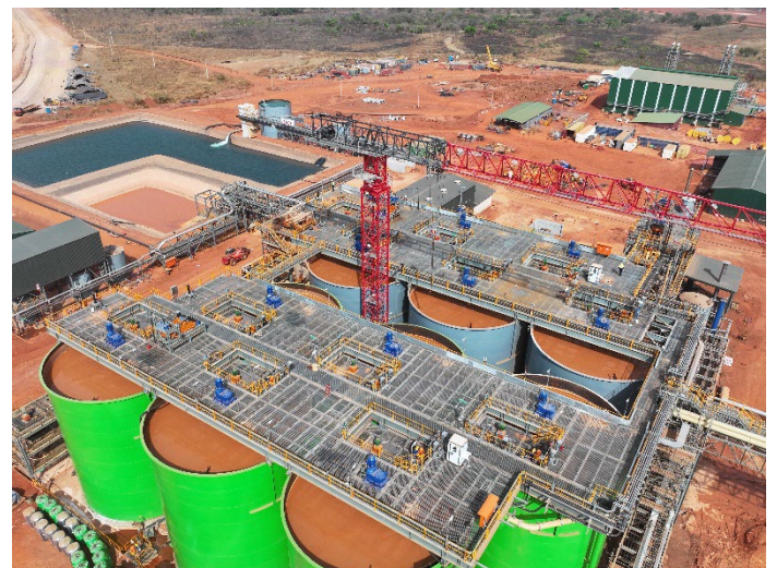
Figure 6: CIL Tank Train A & B
