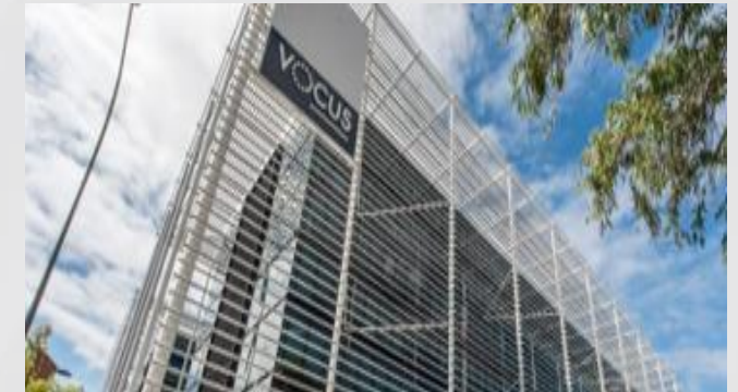
WorkZone West, Perth | $92.0m
