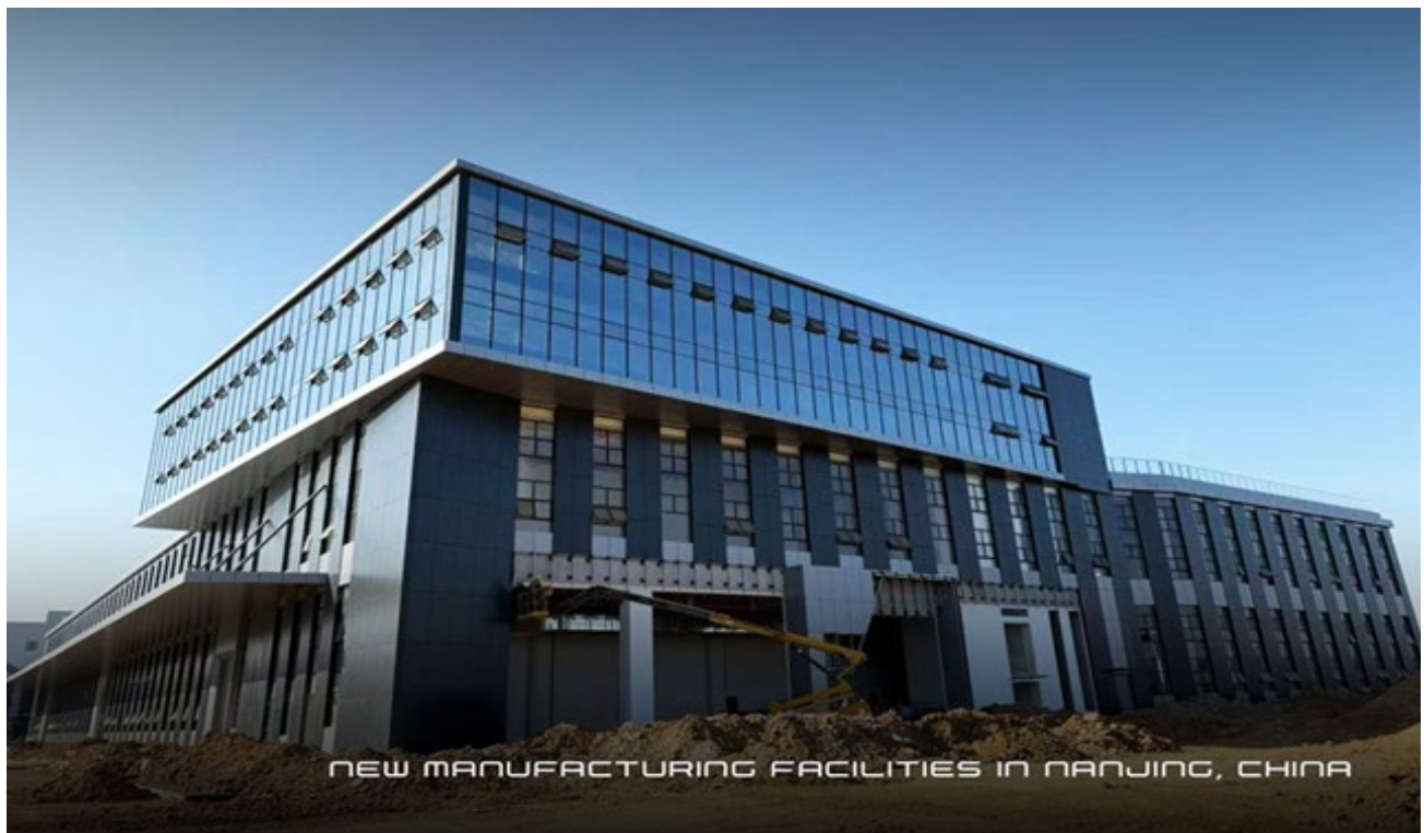
Photo: Vmoto's new manufacturing facilities in Nanjing, China.
