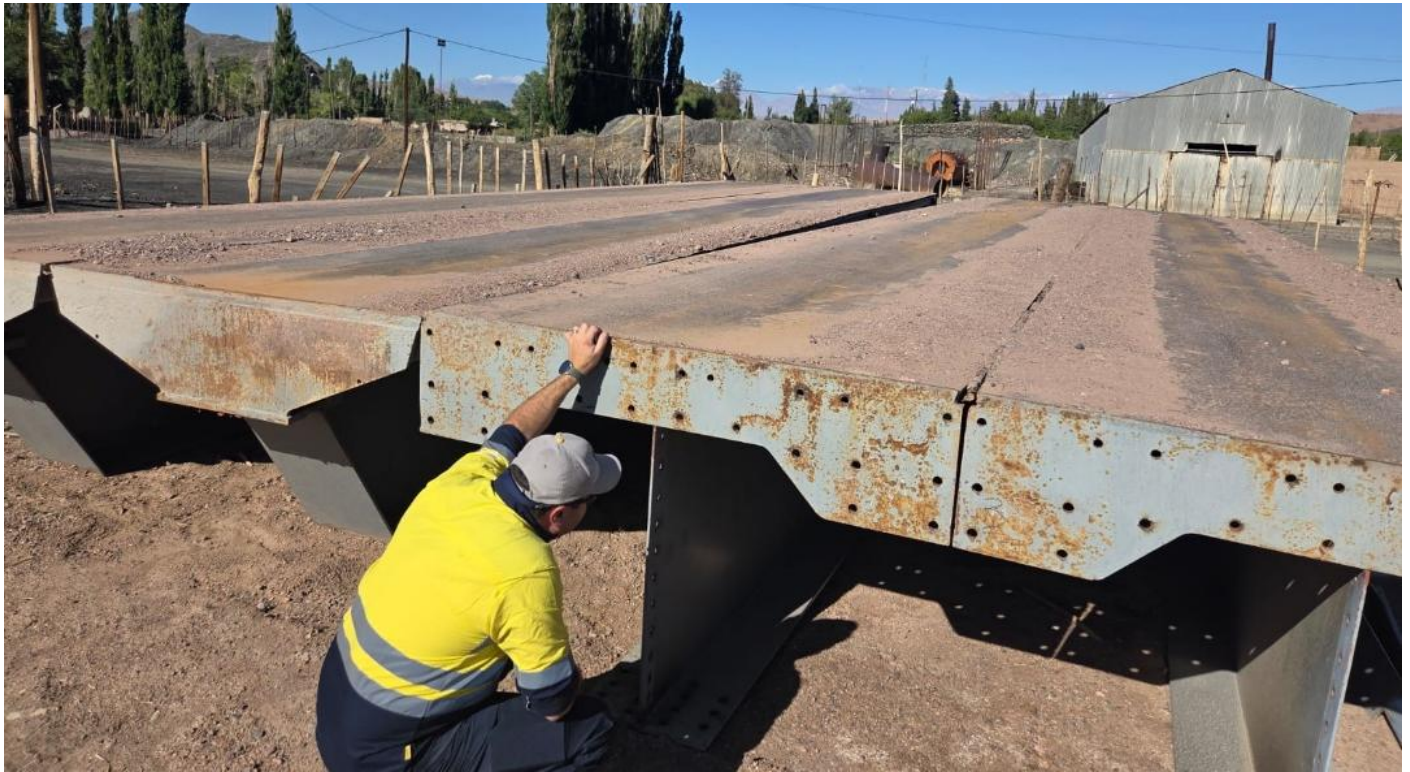
Figure 6 - Bailey Bridge Module Segments Inspection
