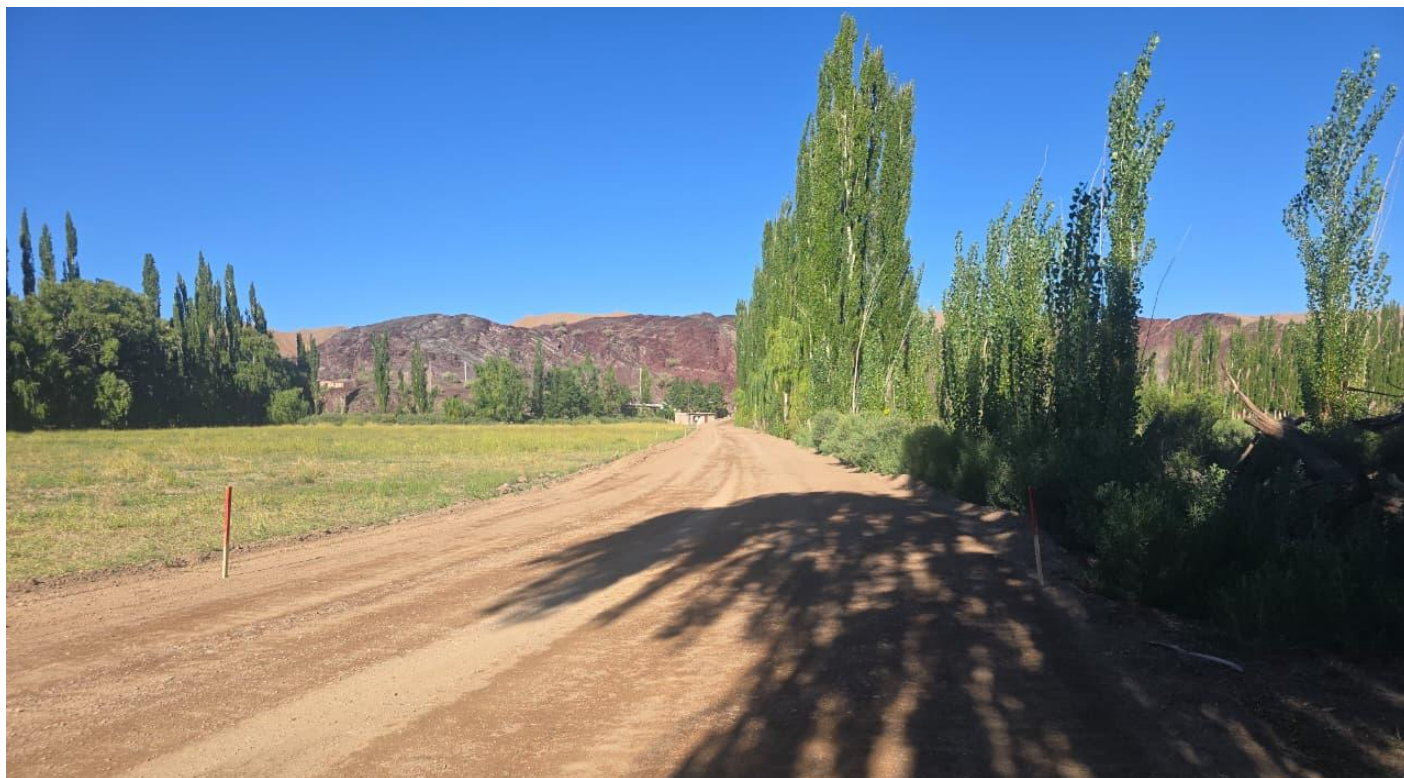
Figure 3 – Completed segment of Calingasta Bypass Road
