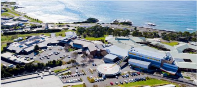
Northwest Private Hospital – Stage 2 Location: Regional, TAS | Approx Value : $15m
