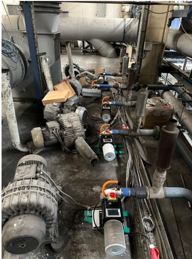
Image: 22kW side channel blowers replaced by 7.5kW Sprintex G15
