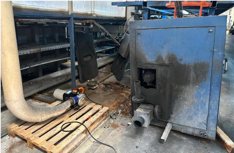
Image: Installed Sprintex G15 (left) compared to removed legacy Roots blower (right)
