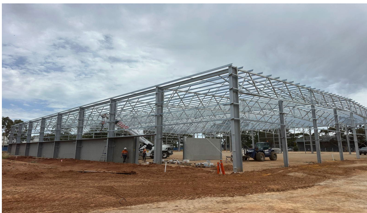
Image 5: SA1 Salisbury Bioenergy Project construction
