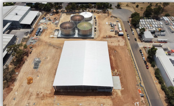
Image 9: SA1 Salisbury Bioenergy Plant Construction
