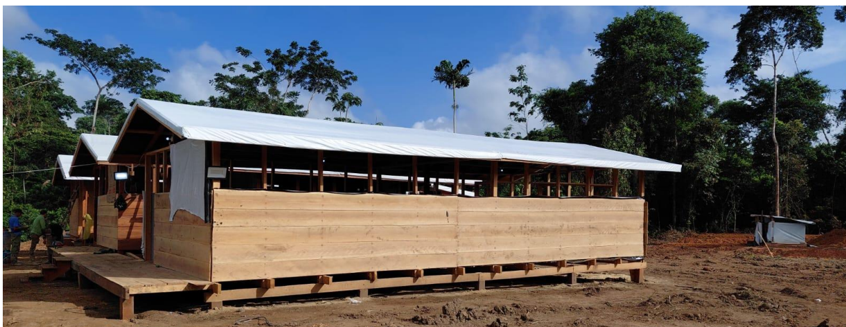
Figure 12: SOKO trench camp progress in early February.
