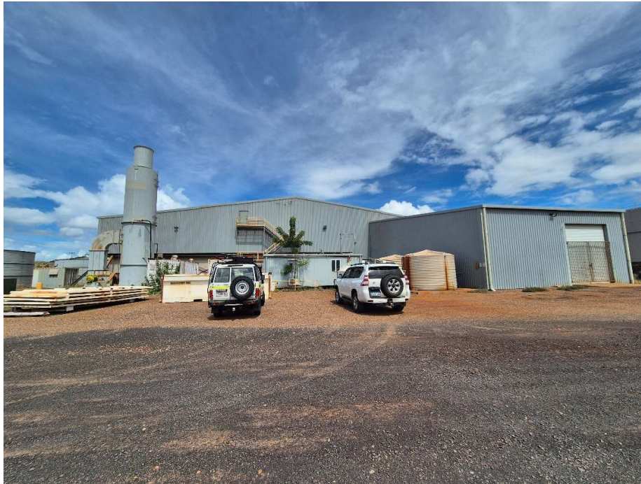
Figure 5: Concentrate Shed at Wyndham Port
