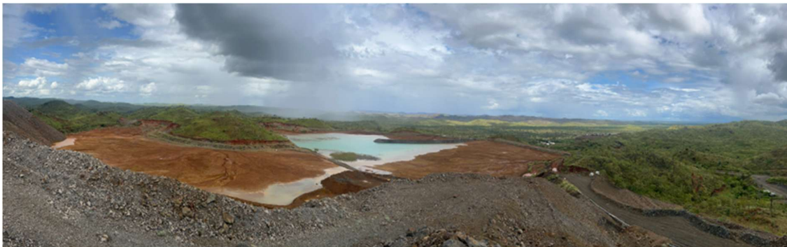
Figure 4: Savannah Tailings Storage Facility
