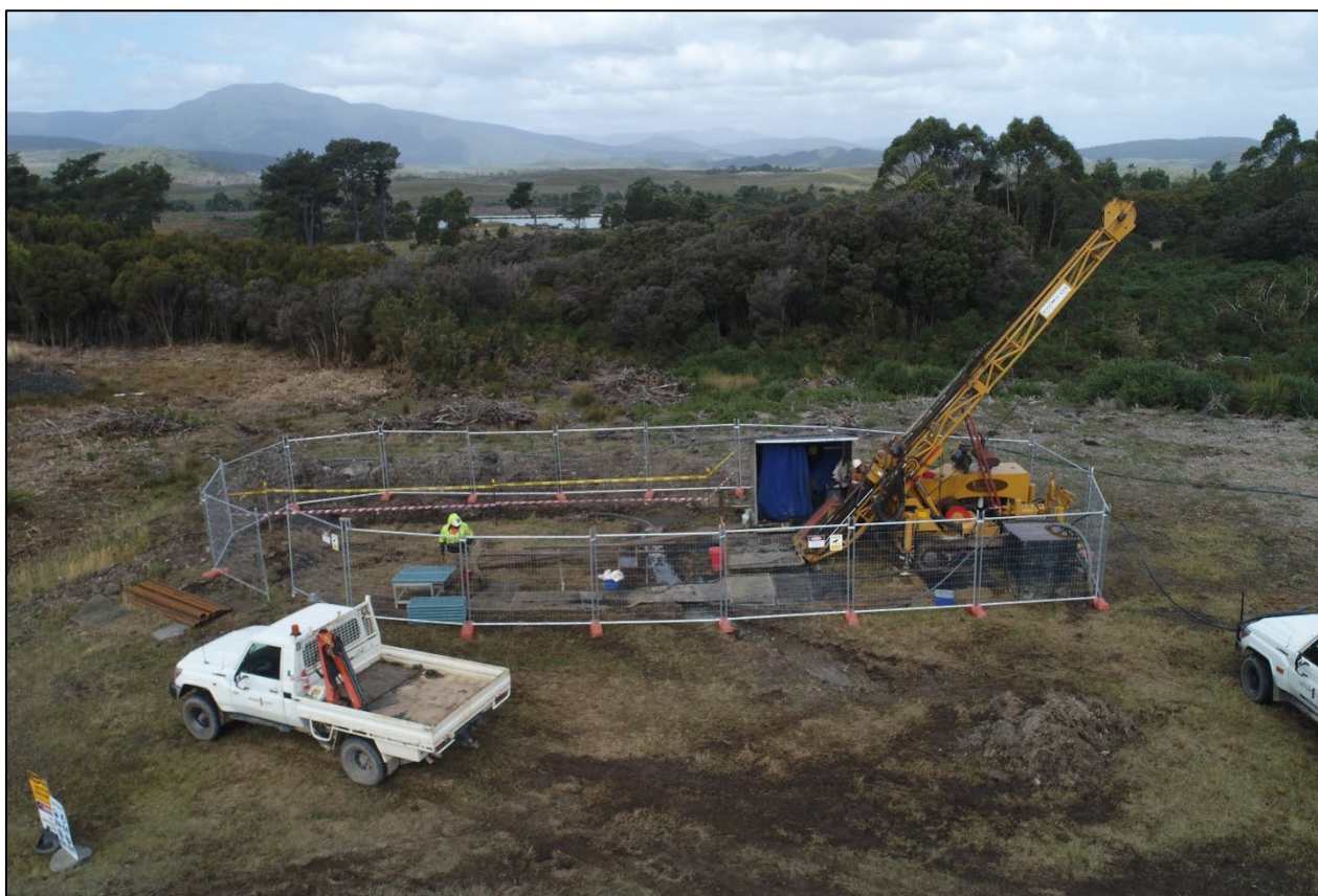
Figure 4 - Drill Rig on site at Silver King Prospect
