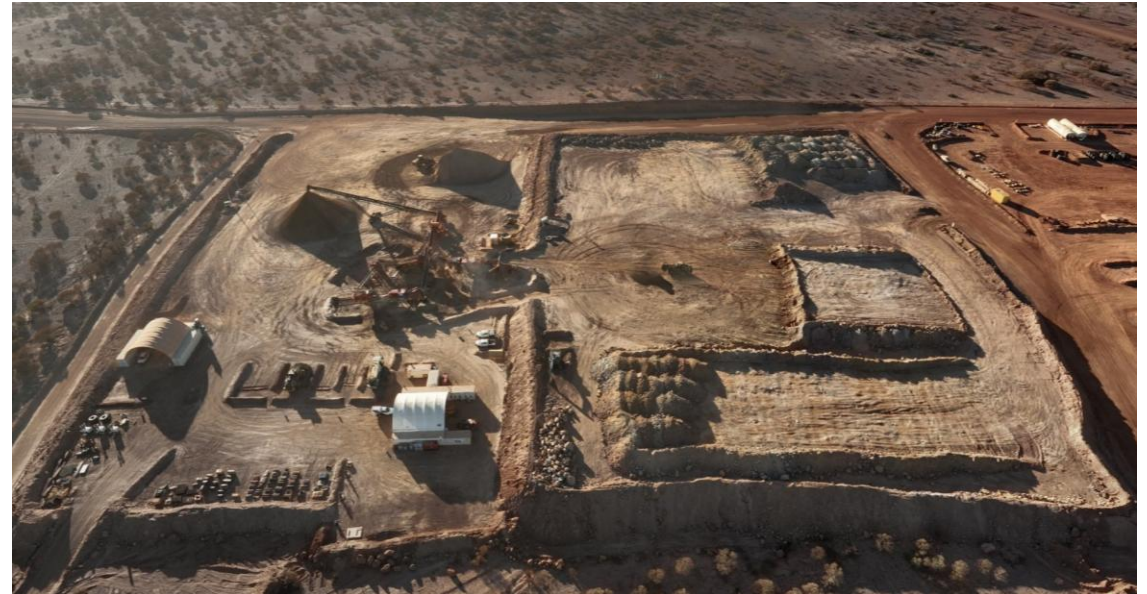
CP ROM and Crusher Pad 31 January 2026
