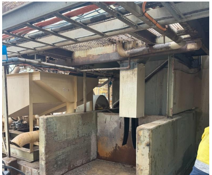
Figure 4: Mill steel work scats shoot install
