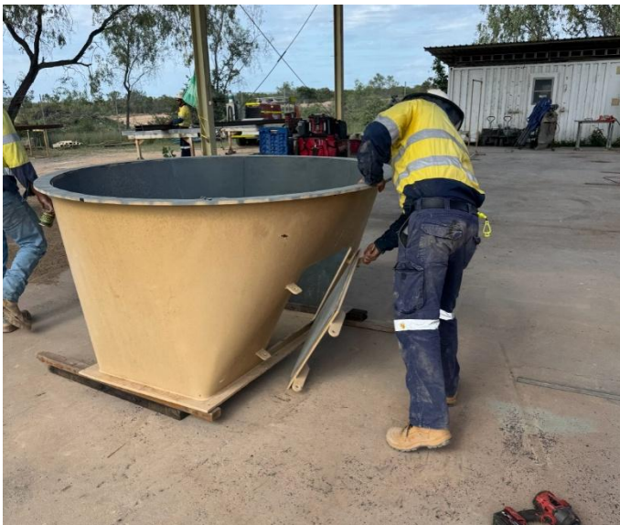
Figure 3: New Fine Ore Bin Chute Replacement
