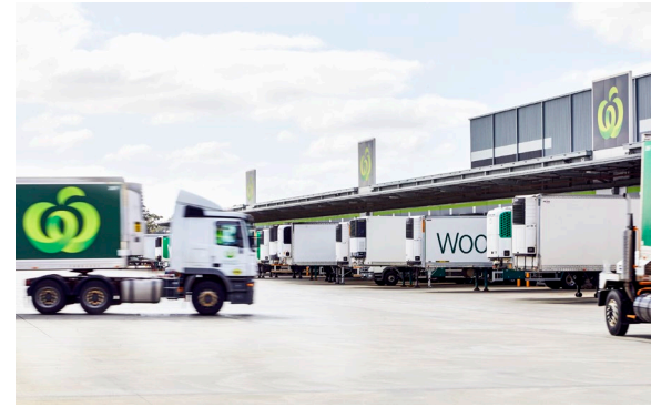
Woolworths Distribution Centre, Melbourne
