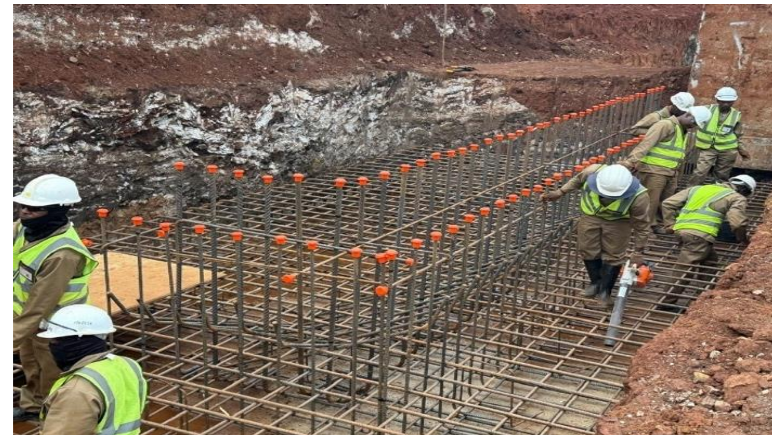
Retaining wall steelworks
