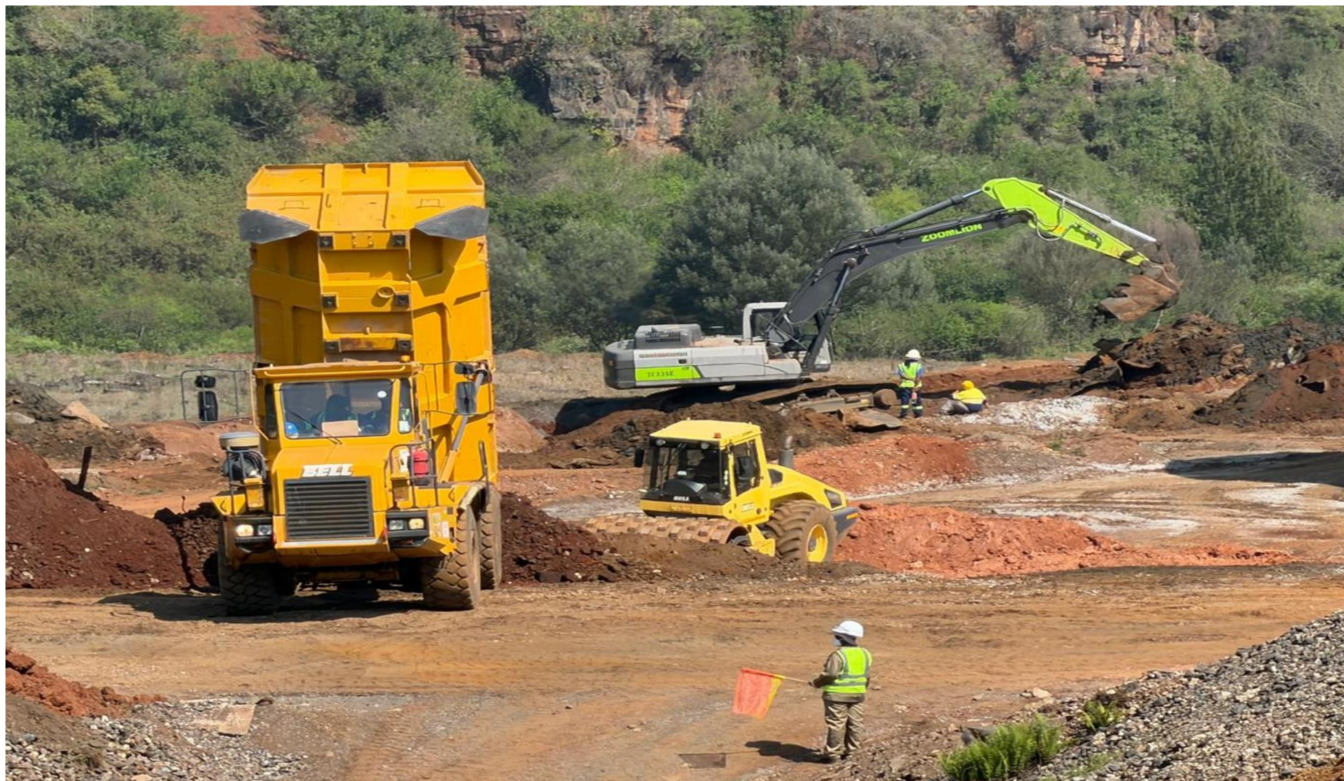
Earth works in progress at the Gold plant
