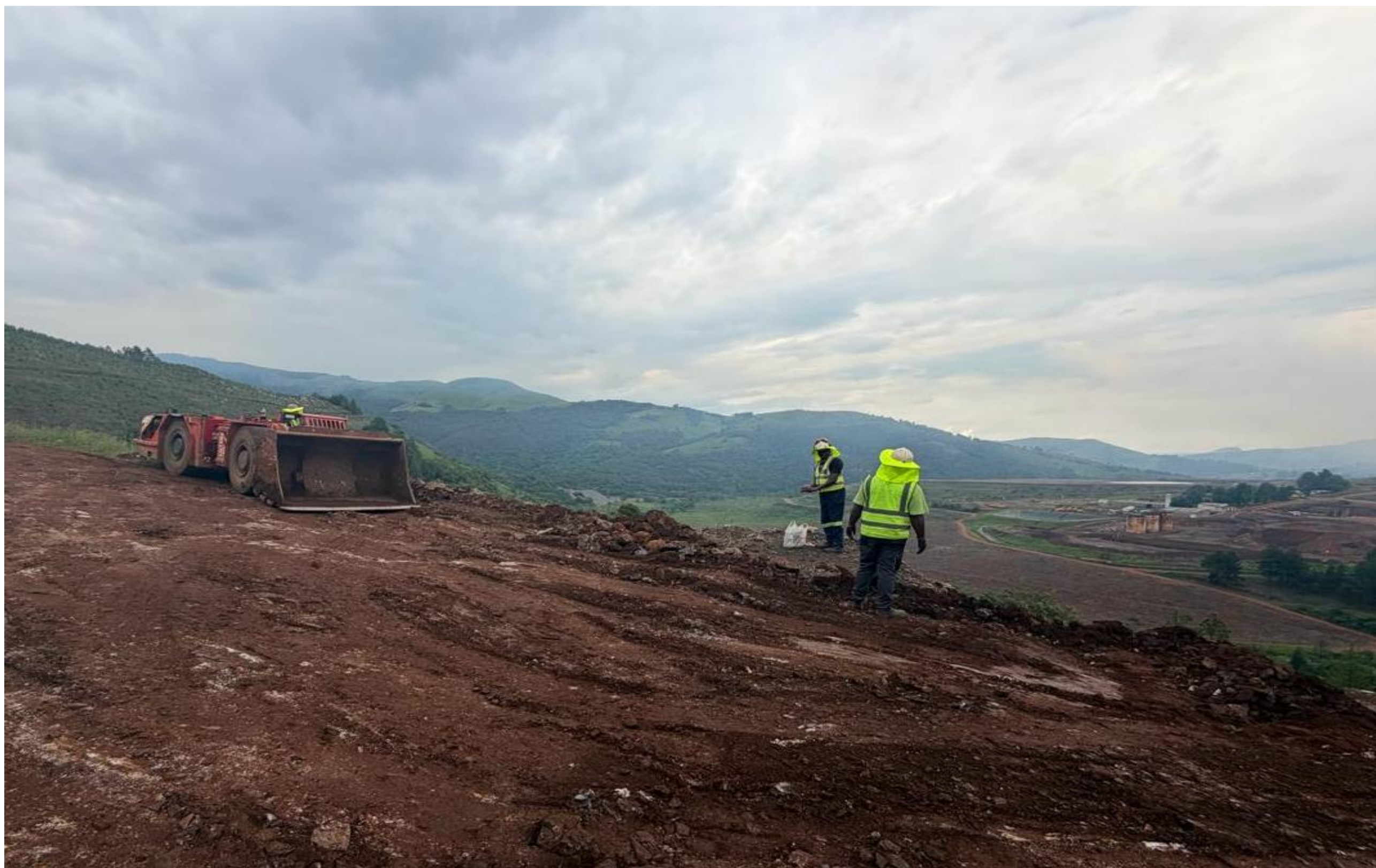
Beta Gold Mine access road under construction
