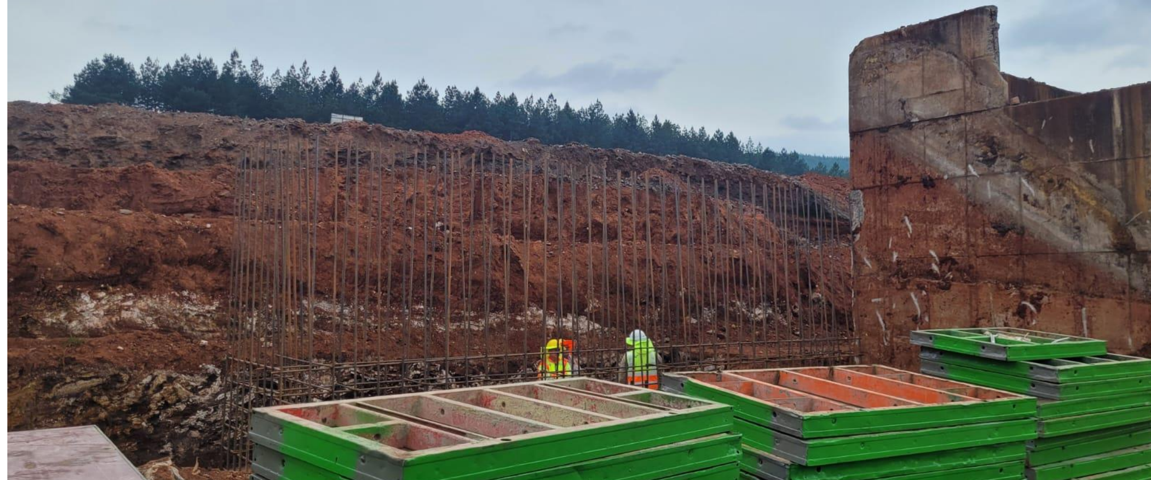
Terrence 2 Foundations and formwork
