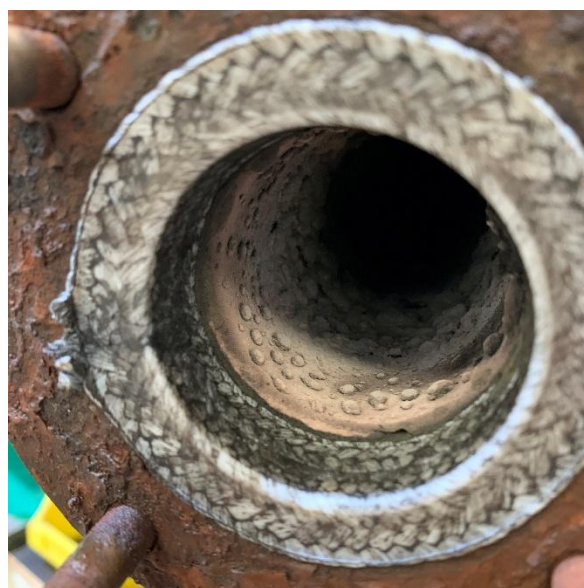
Figure 3. Reactor tube with condensed HCl
