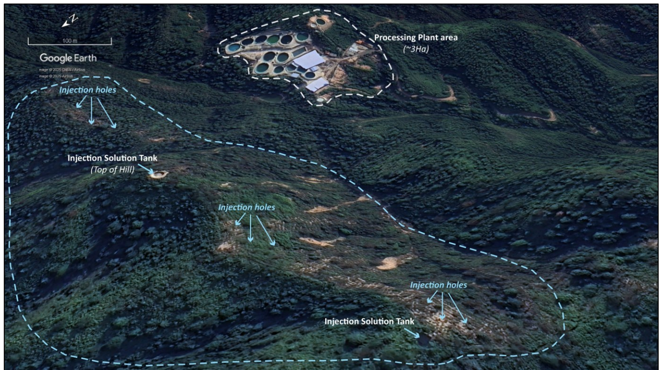
Figure 6. Google Earth 3D view of an ISL rare earth operation in Jiangxi Province, China, showing hill-slope leaching areas feeding a hydrometallurgical processing plant.
