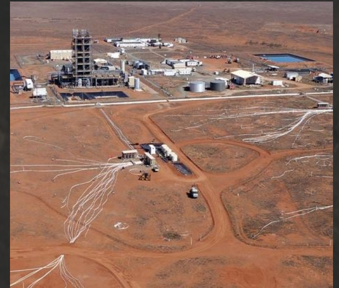
Boss Energy Honeymoon Operation
