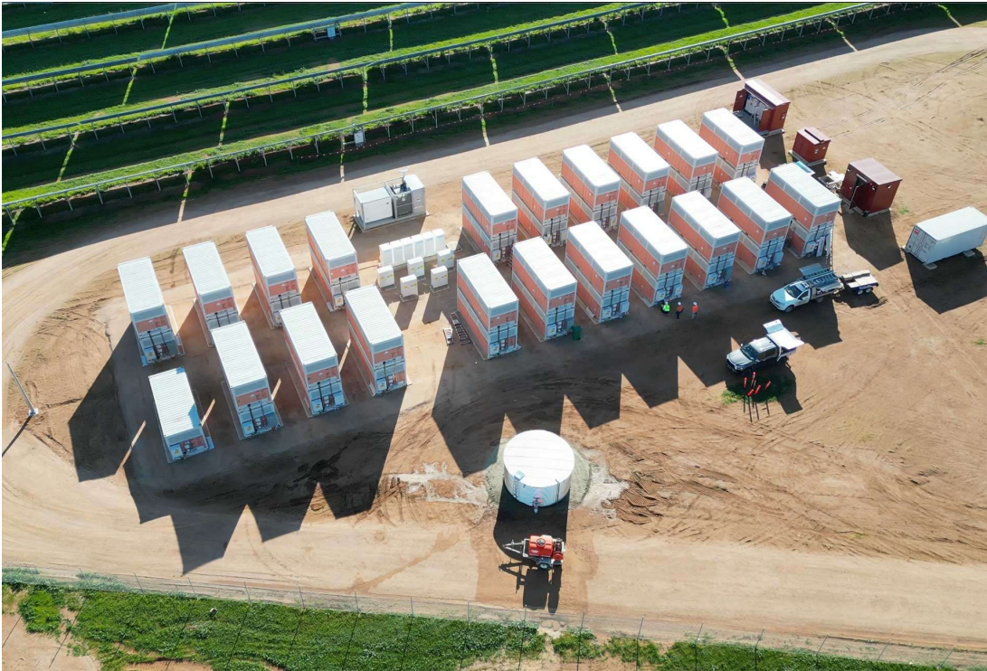
Figure 1. Example VFB installation (Yadlamalka Invinity 8 MWhr VFB )
