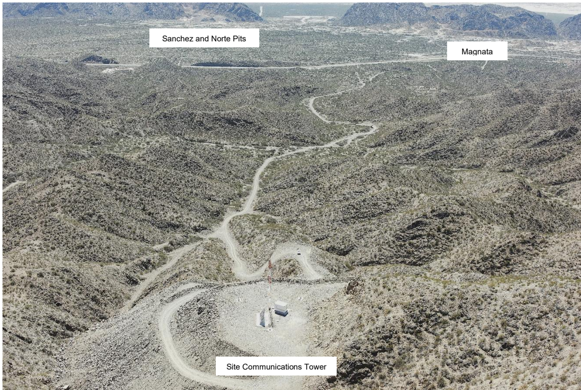
Figure 6 - Communications Tower looking back to Hualilan as at 17 December 2025
