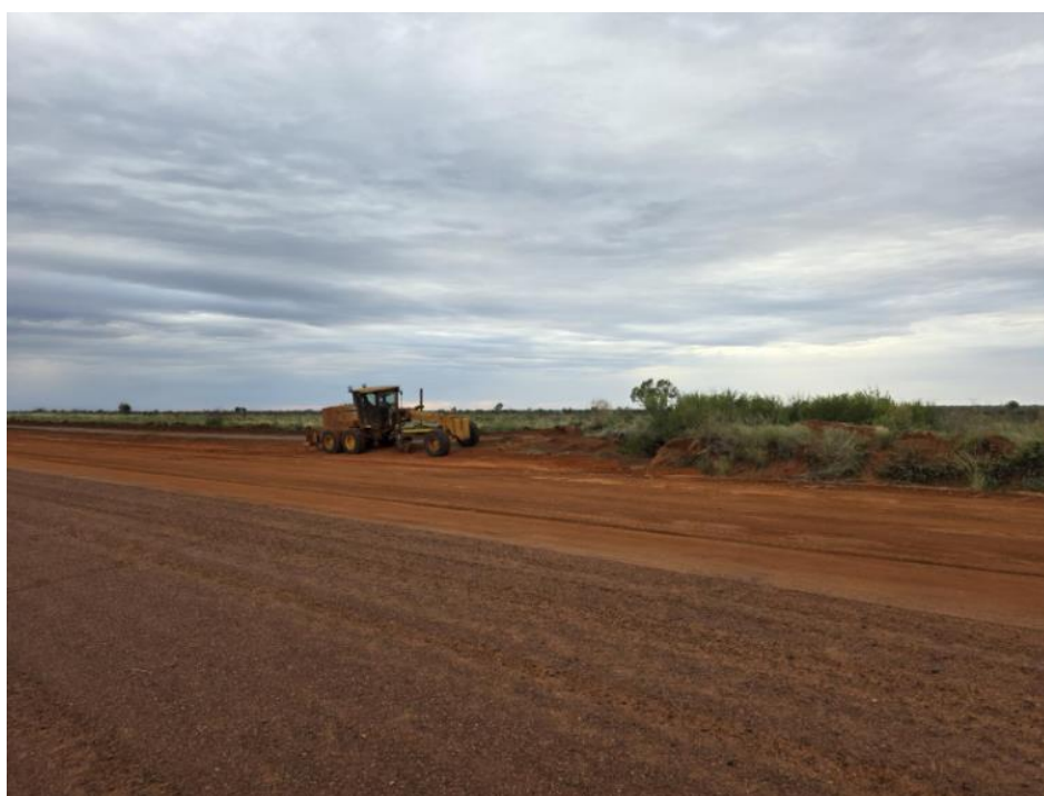
Figure 3: Airstrip compliance and conditioning works
