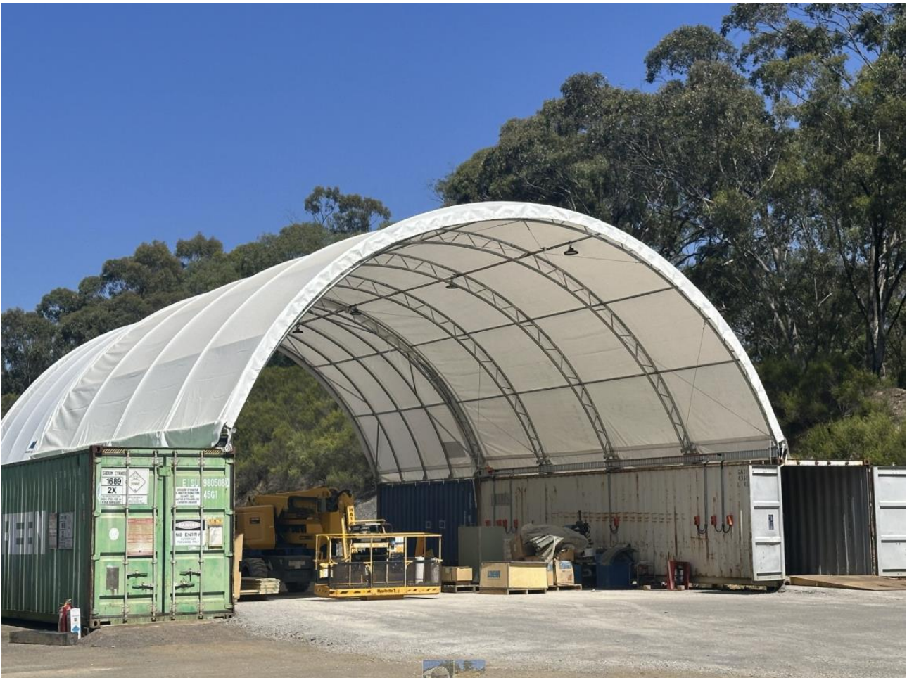
Figure 10. New Heavy Fabrication Workshop
