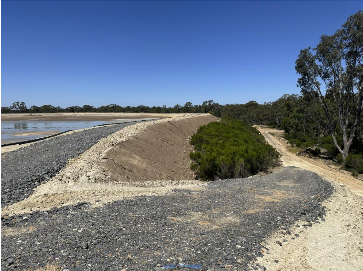
Figure 12. Tailings Storage Facility lift 5 D completion
