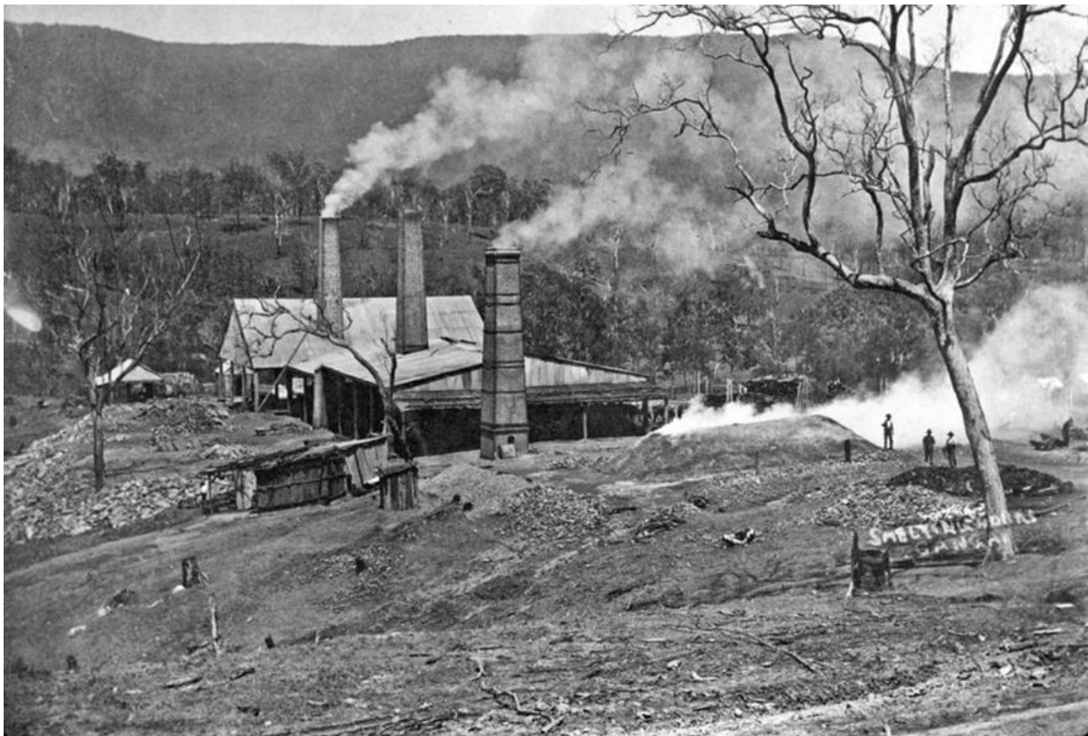
Figure 3: Historical smelting furnaces at the Cangai Copper Mine
