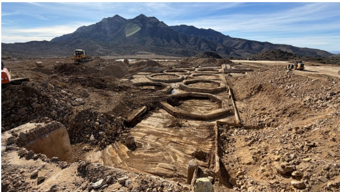
Figure 3: Uncovered concrete structures at Colosseum 5
