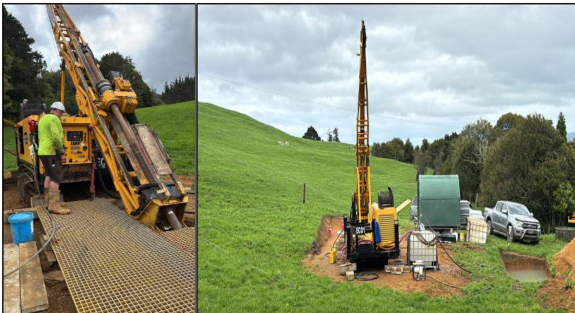
Figure 1: Drilling the first hole at Scotia South, Waitekauri Gold Project
