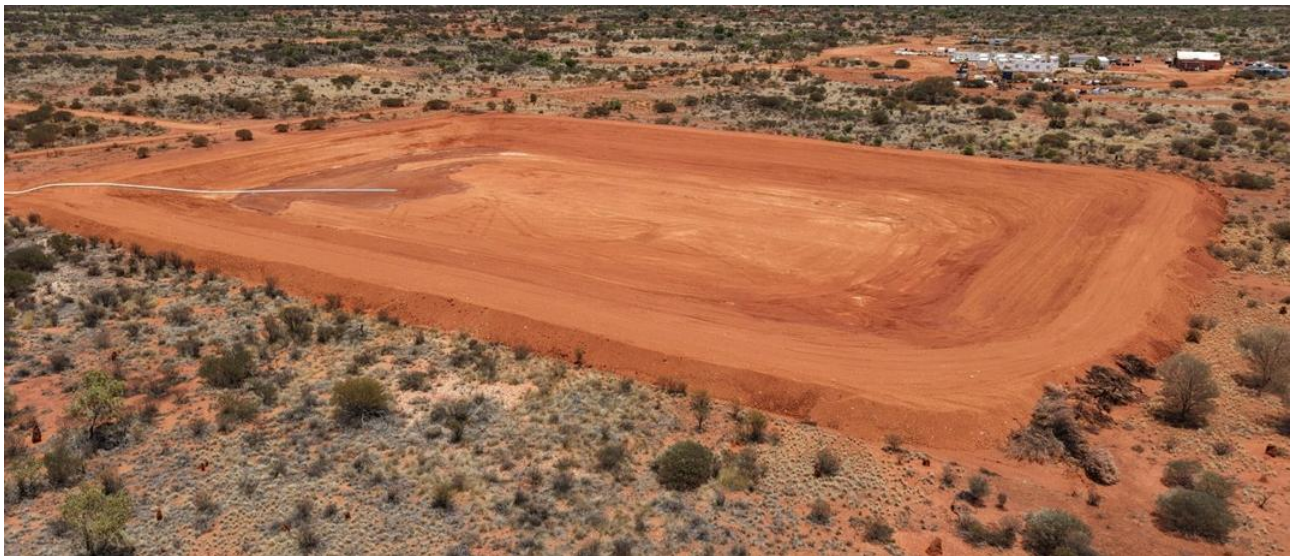
Figure 4: Water-containment sump for the commencement of long-term pump testing
