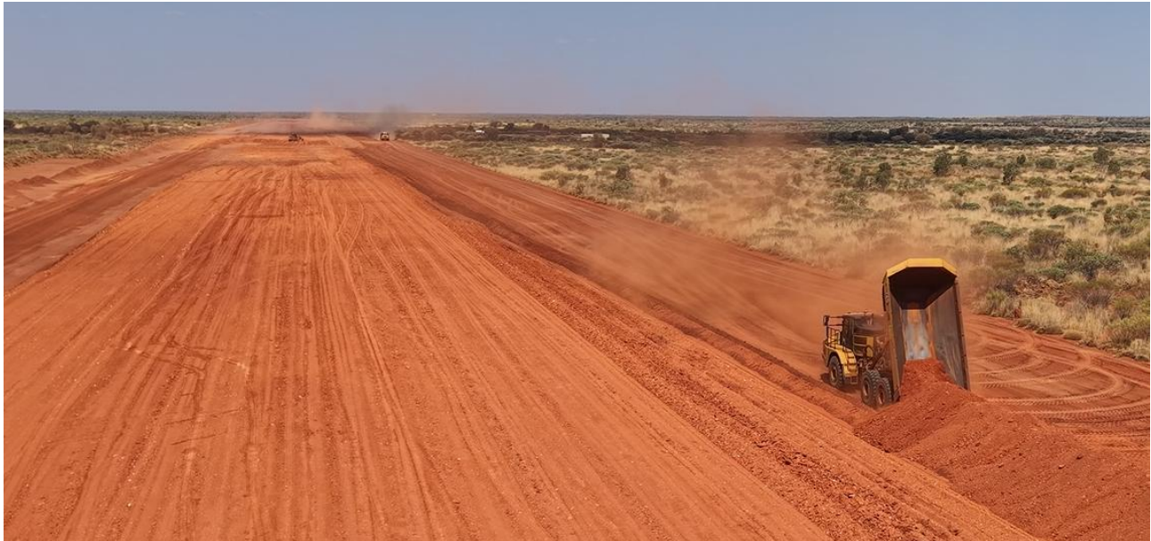
Figure 3: Construction of airstrip in progress
