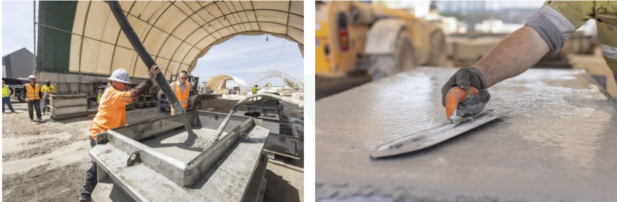
Figure 3 & 4: Wind farm concrete trials - 50% AusPozz™ mix design
