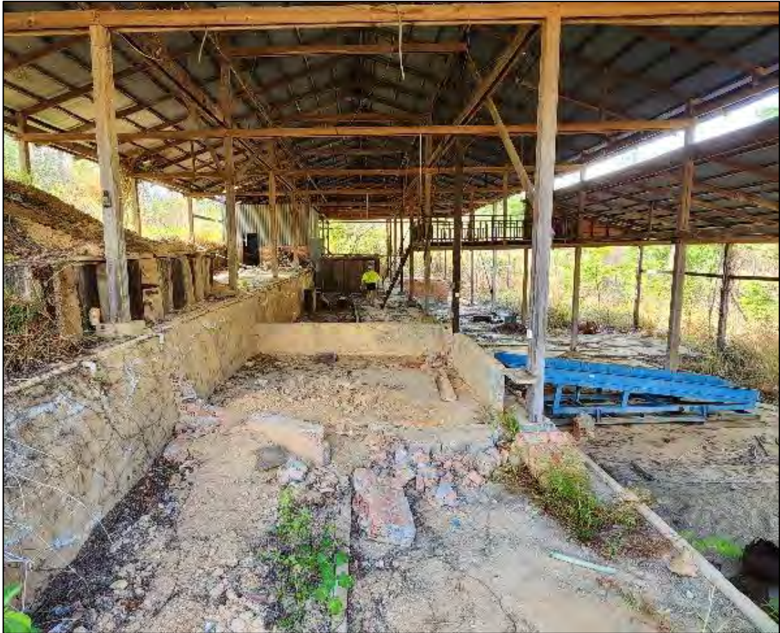
Photograph 6. GMG ore treatment plant located within the O'Phlay Licence in 2024. The GMG plant was closed down in approximately 2020 by the Cambodian government and now lies in ruin.
